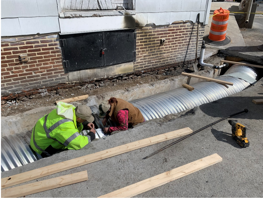
Figure 5: Installing the new culvert (03/17/2020).
