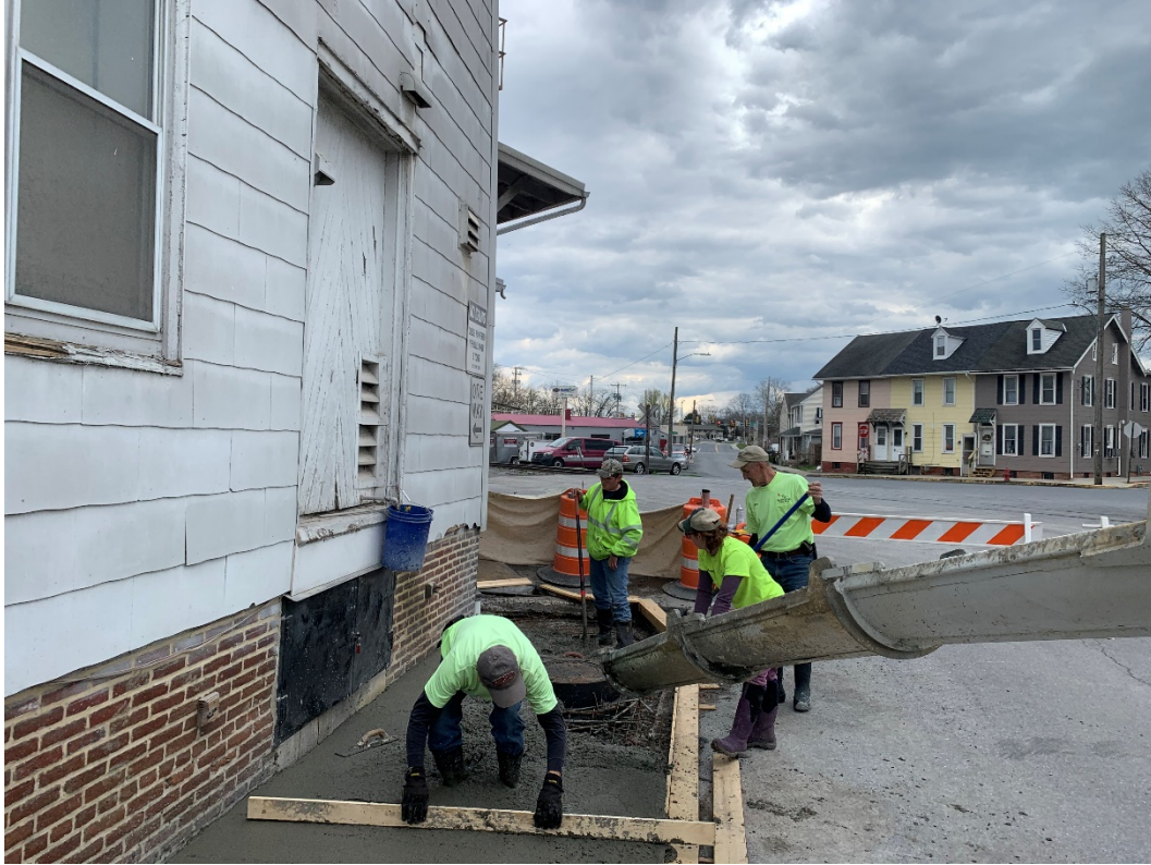
Figure 7: Pouring the new concrete sidewalk (03/30/2020).
