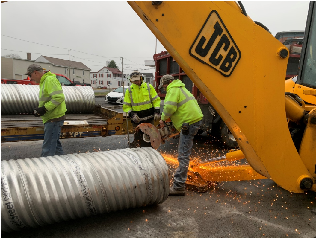
Figure 3: Preparing the new culvert for installation (03/17/2020).
