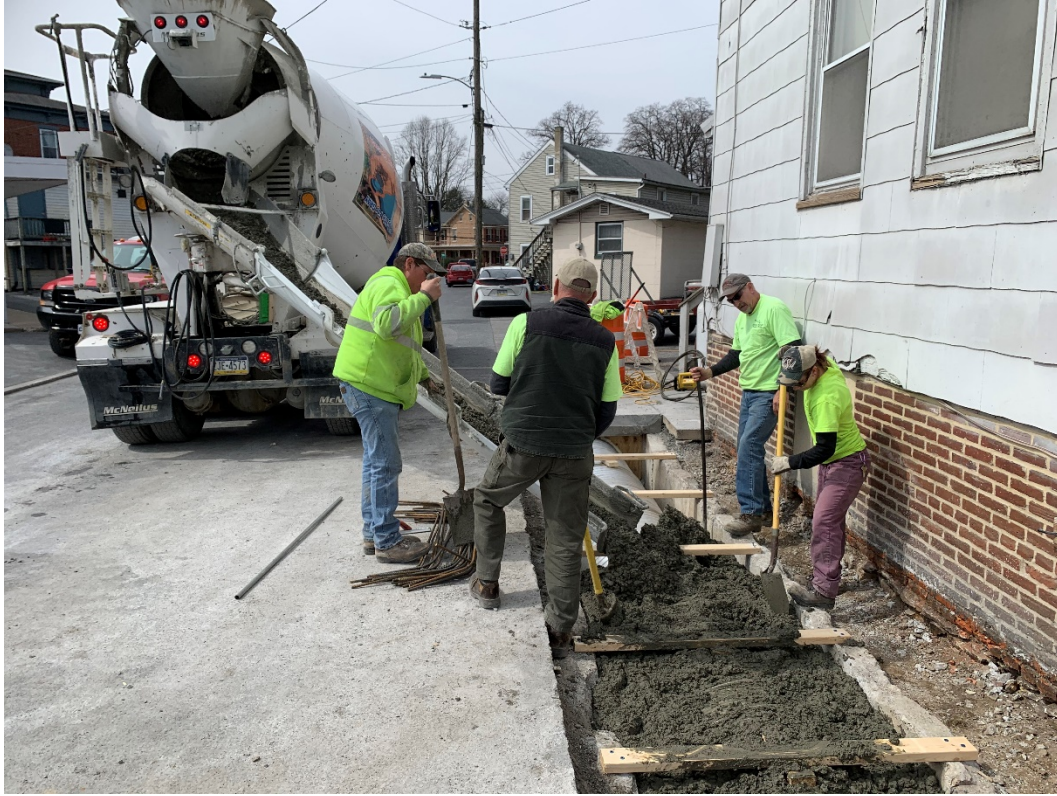
Figure 6: Pouring concrete around the new culvert (03/18/2020).
