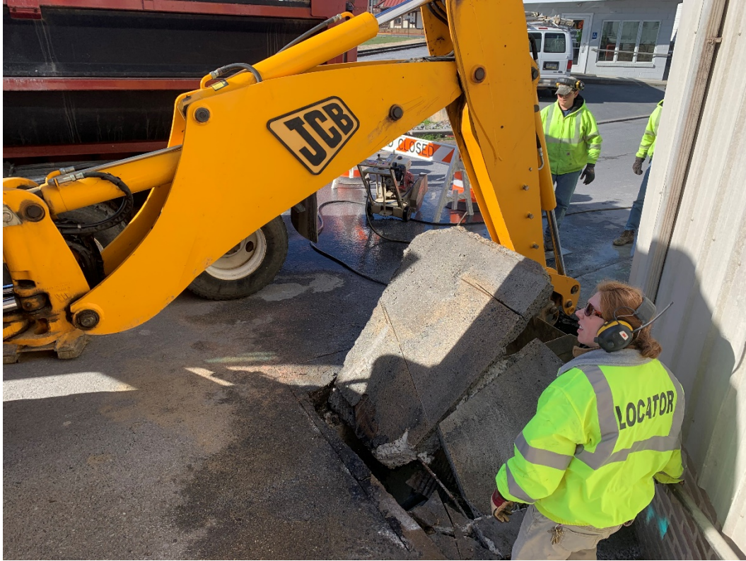
Figure 1: Excavation of deteriorated culvert at New Charlotte Street (03/16/2020).
