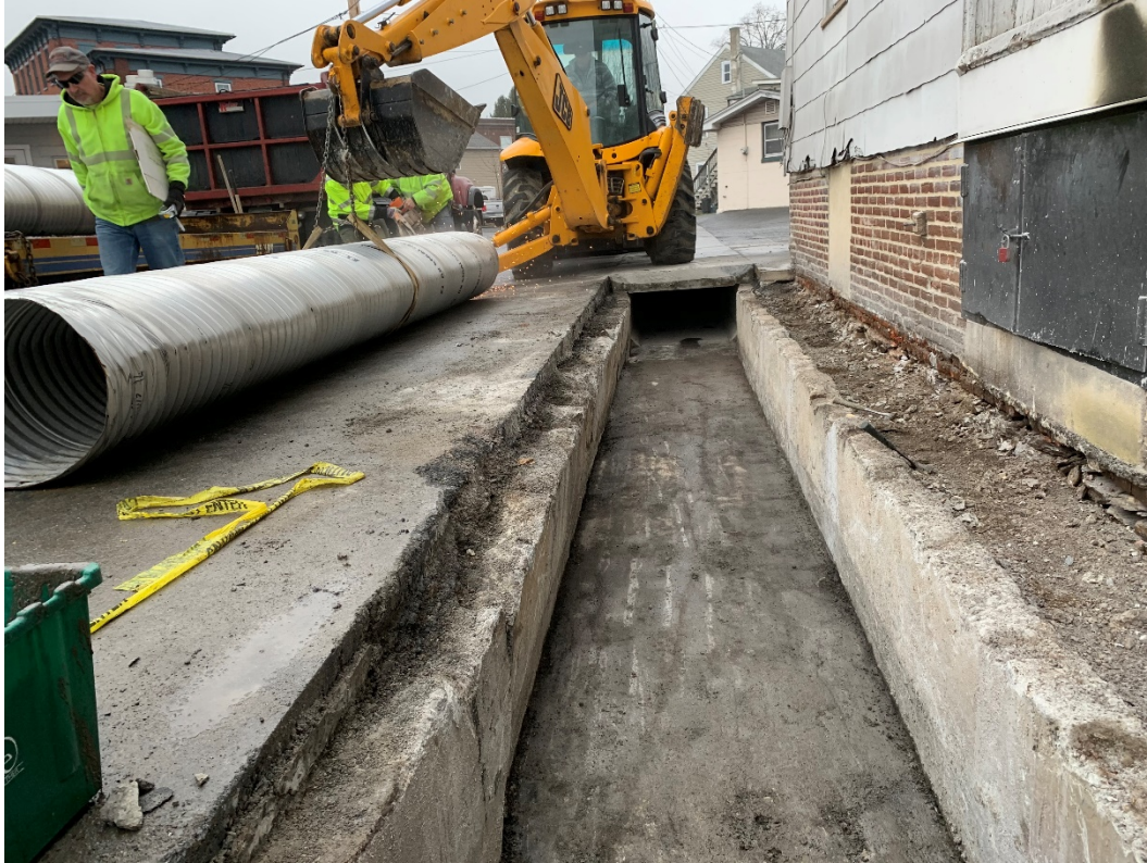
Figure 2: Top slab of existing culvert has been removed (03/17/2020).
