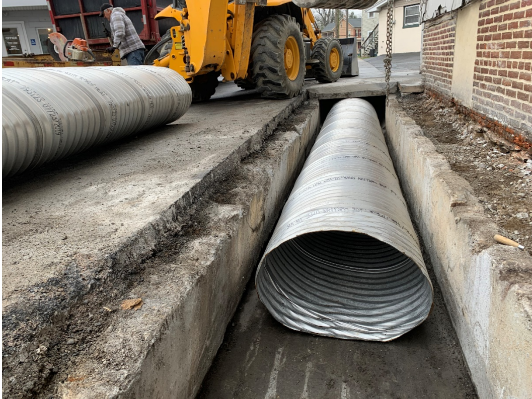
Figure 4: Installing new culvert (03/17/2020).
