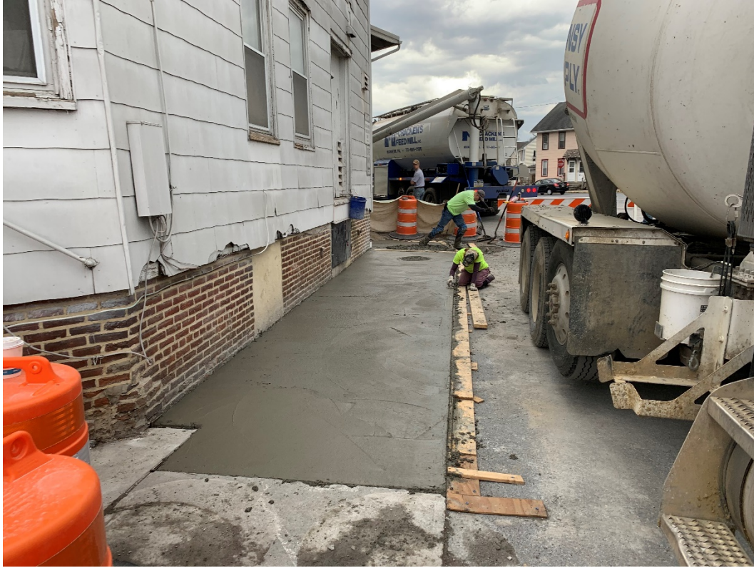
Figure 8: Finishing the concrete sidewalk (03/30/2020).
